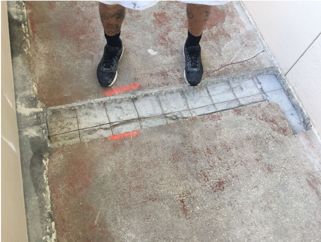
Picture 1: Topping repair at panel butt joint
